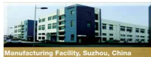
Manufacturing Facility, Suzhou, China
