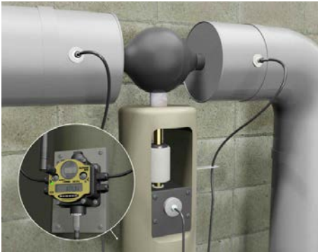
监测压差，确定更换滤芯
