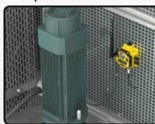
A Banner Wireless Node, is used to activate a pump that could be used for direct irrigation or to fill a tank. If the radio link is lost for any reason, the Node outputs can be configured to stop automatically and send an alarm to key personnel.
