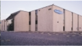
Banner Manufacturing Plant Minneapolis, MN USA
