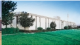
Banner Manufacturing Plant Aberdeen, SD USA
