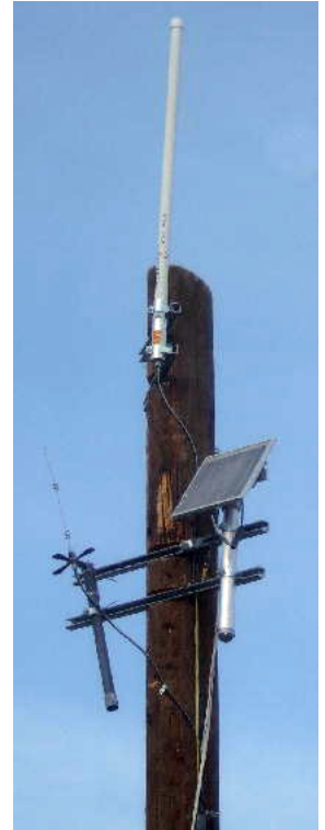
Data radio and Gateway (used as a repeater) and powered by a solar panel.
